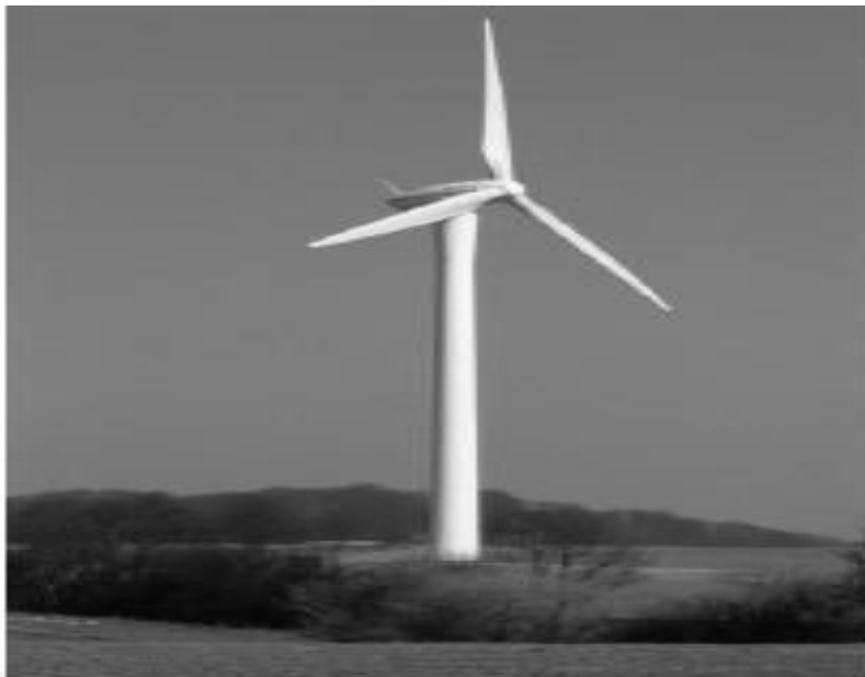
Wind Turbine Generator units
