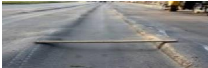
Fig.6: Real-Time Formation of Ruts
